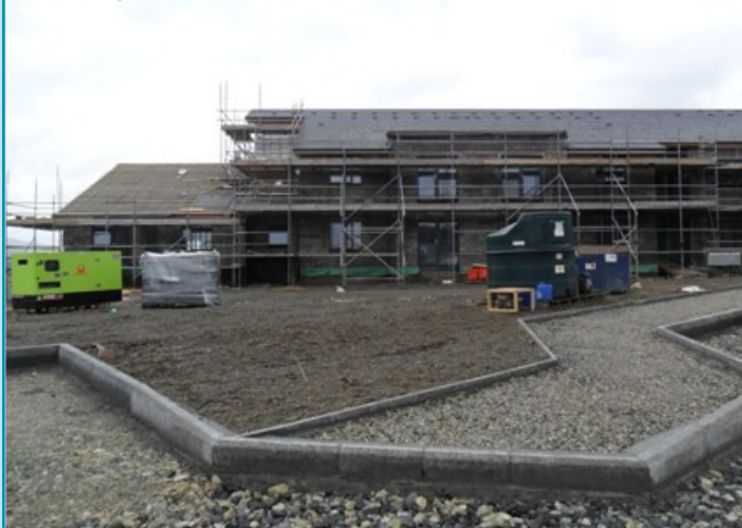
Mull Progressive Care Centre under construction
